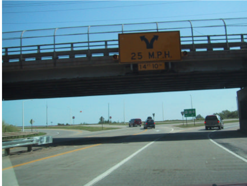
Photo 3-4: Front Street and US-41/M-28 Intersection
