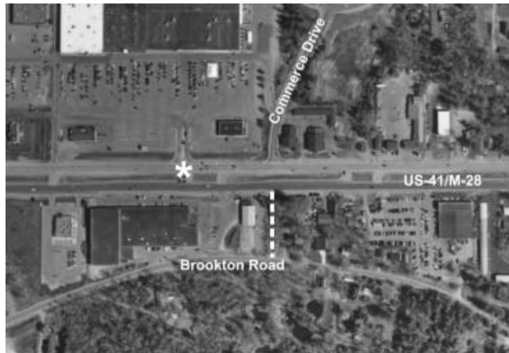
Photo 3-16: Westwood Mall Traffic Signal (*) and Commerce Drive
