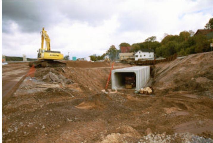
Photo 4-17: Pedestrian Tunnel Under Construction in Houghton
