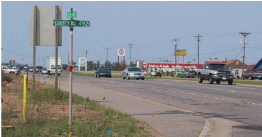
Photo 4-15: Raised Curbs Instead of Sidewalks
