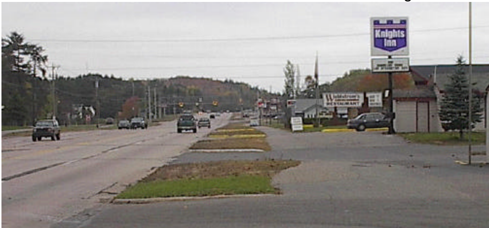
Photo 4-14: US-41/M-28 at Wahlstrom's Restaurant looking north
