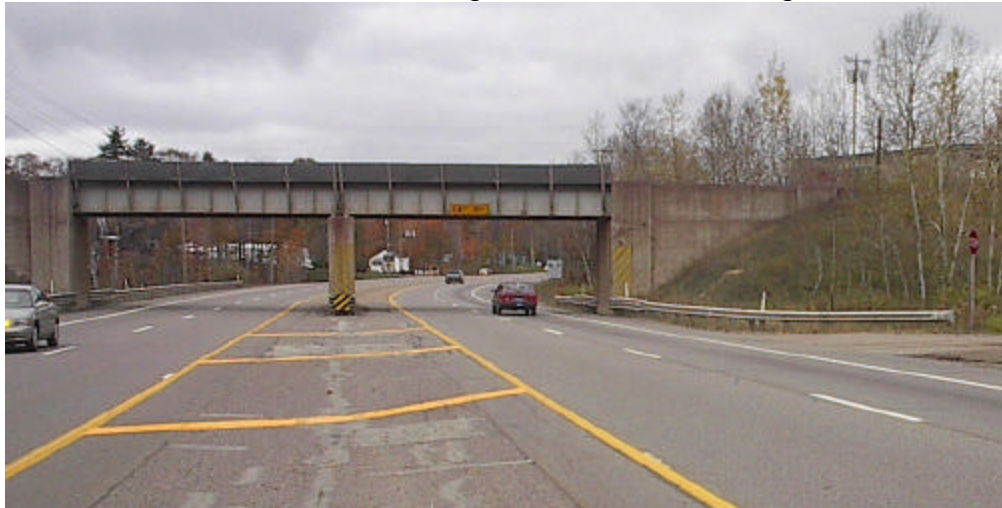
Photo 4-6: Existing 14' Railroad Crossing
