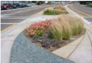
Green infrastructure for visual appeal
