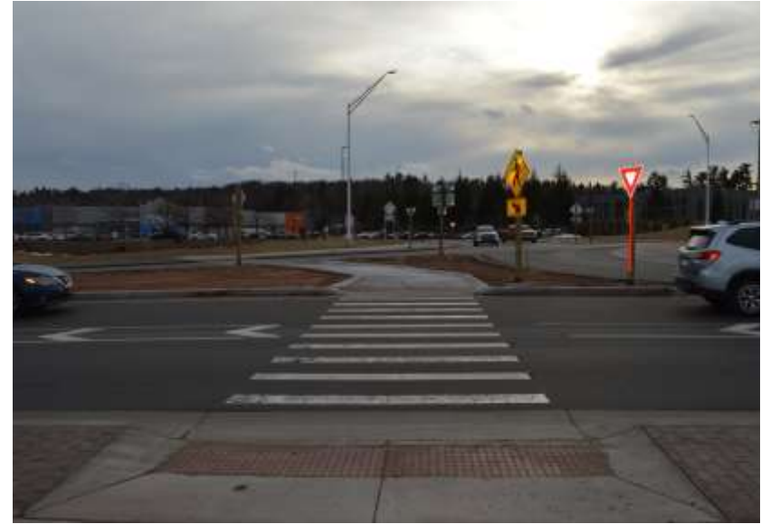
Recently installed roundabout at Co Rd HQ and U.S. 41/M-28
