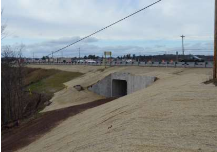
Newly constructed underpass below the corridor
