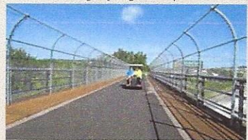
Soo Line Bridge, Marquette
